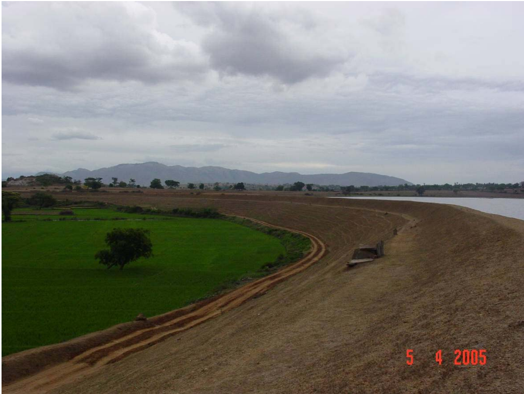
Figure 3-17. A view of the Baragi irrigation tank bund, with the irrigated area on the left.
