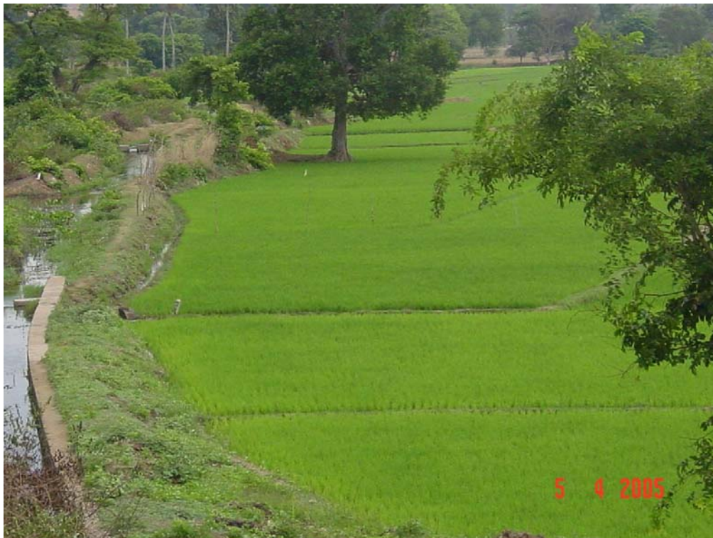
Figure 3-18. A view of the Baragi tank irrigation channel and irrigated area planted with paddy.
