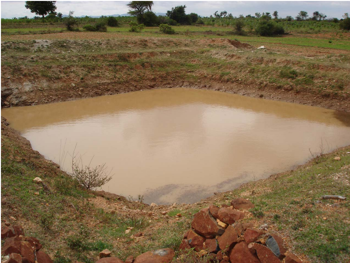
Figure 11. Example of farm pond in good condition (Virupakshapura village, Tumkur district, IWDP programme)
