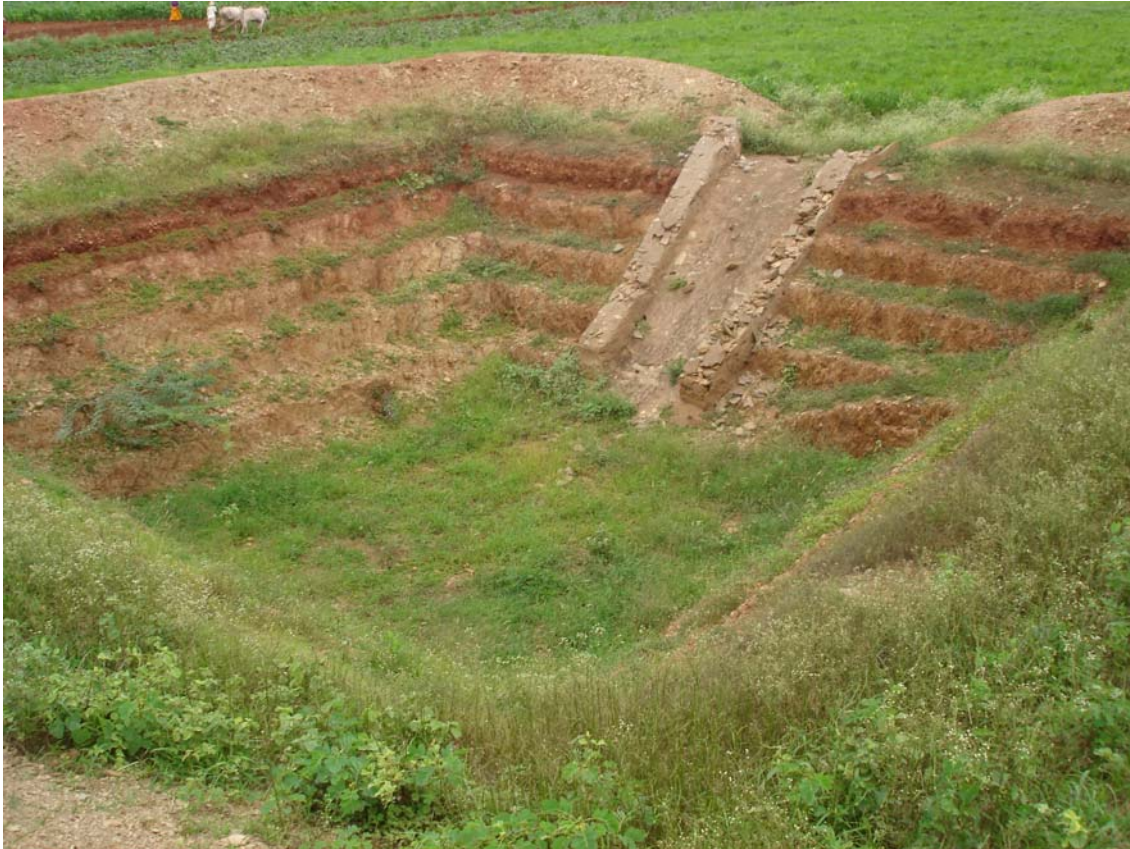
Figure 12. Example of farm pond in poor condition (Guttala village, Haveri district, SUJALA programme)
