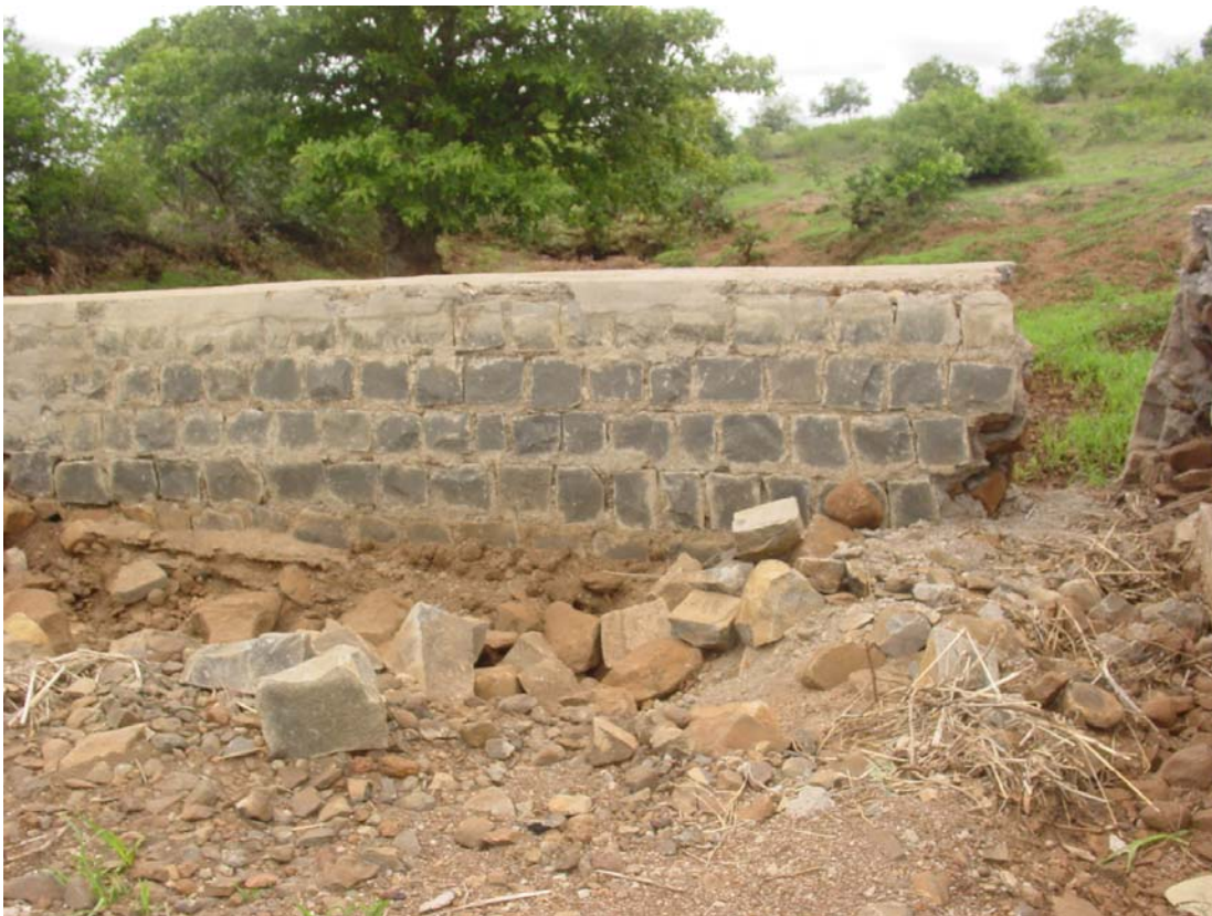
Figure 4. Example of breached check dam (Dongargaon village, Gulbarga district, DPAP programme)
