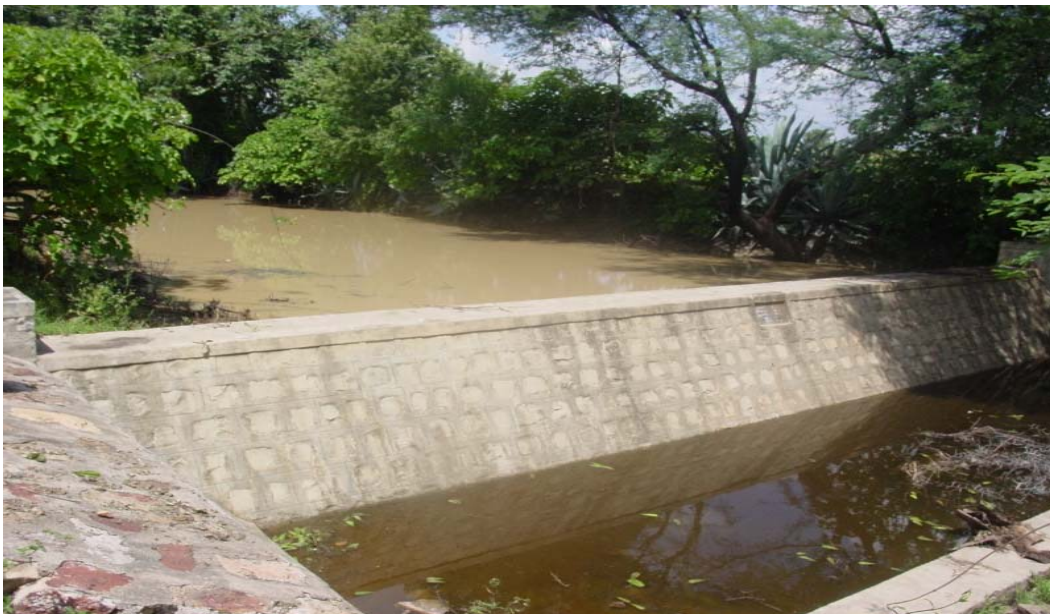
Figure 5. Check dam in 'good' condition: Kalliguddi village, Belgaum district, DPAP programme
