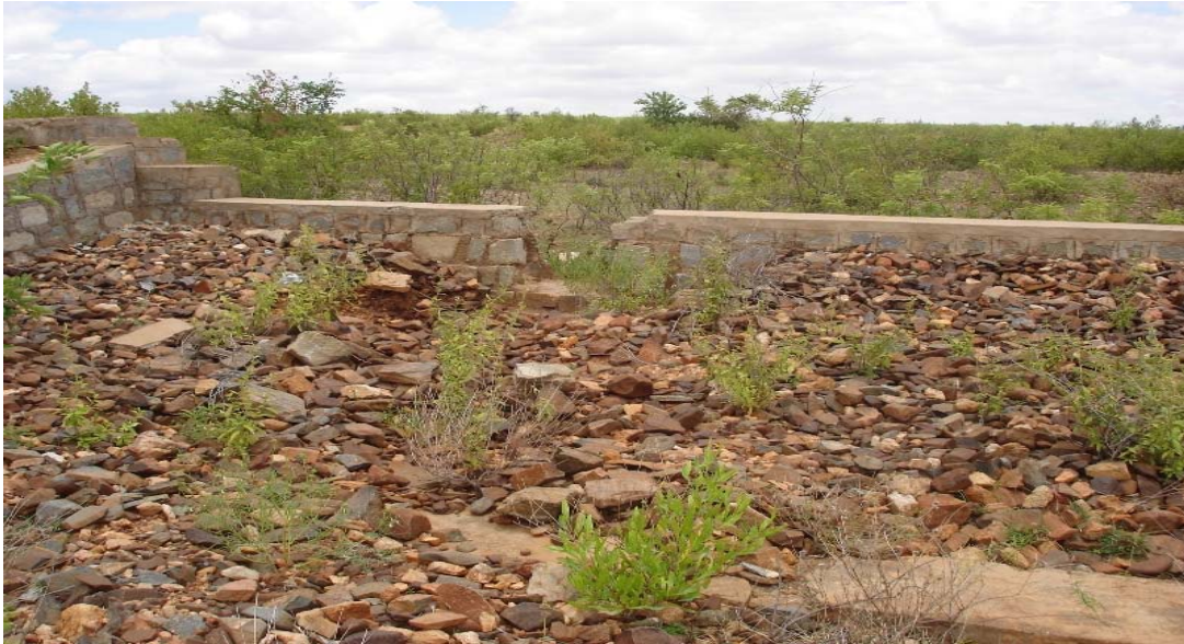
Figure 3. An example of check dam in poor condition—in Maddihalli of Hiriyur taluk under NWDPRA programme
